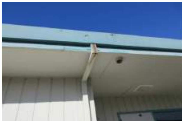
#18 SOFFIT AND DOWNSPOUTS
