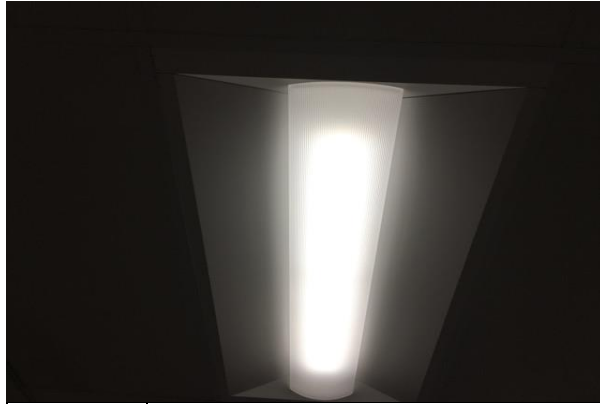
#25 LIGHTING SYSTEM, INTERIOR
