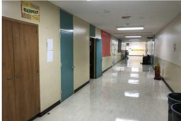
#13 MAIN BUILDING HALLWAY
