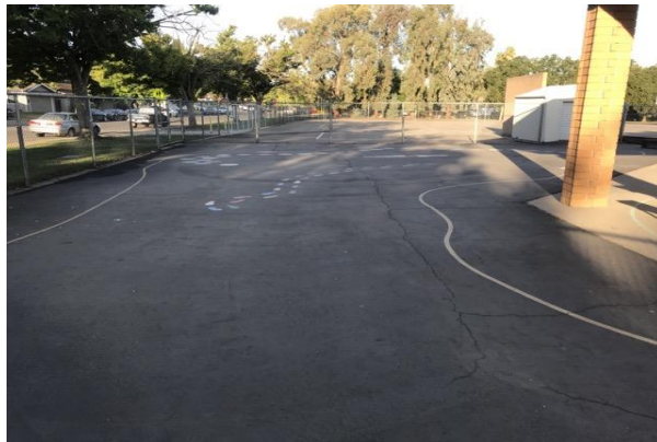
#29 PEDESTRIAN PAVEMENT, SIDEWALK, ASPHALT
