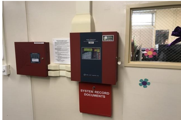
#28 FIRE ALARM CONTROL PANEL, BASIC/ZONED
