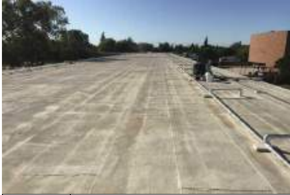
#13 001 A WING, B WING, ROOF, MODIFIED BITUMINOUS
