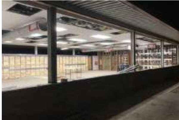
#19 E WING AND F WING CONSTRUCTION
