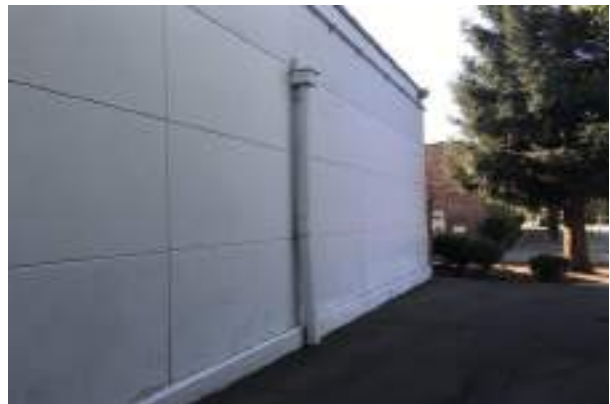
#10 015 CAFETERIA, PAINTED CONCRETE
