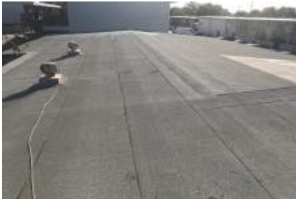
#15 013 ROTC, ROOF, MODIFIED BITUMINOUS
