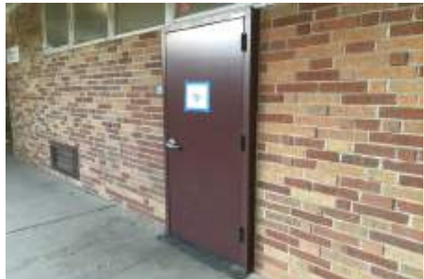
#6 EXTERIOR DOOR, WOOD SOLID-CORE
