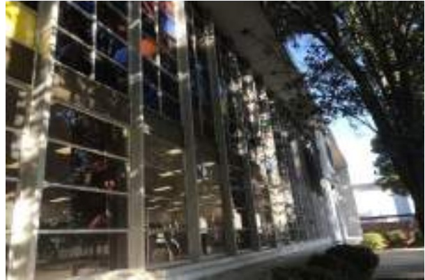
#8 015 CAFETERIA, CURTAIN WALL, ALUMINUM-FRAMED SYSTEM WITH GLAZING
