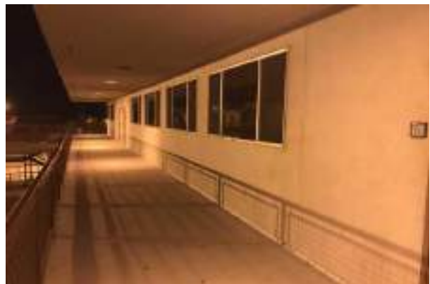
#12 P02 X04-X08, EXTERIOR WALL, STUCCO, 1-2 STORIES
