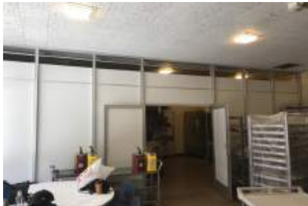
#23 015 CAFETERIA BREAK ROOM, INTERIOR WALL FINISH, PLATE GLASS
