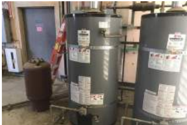
#41 013 ROTC, DOMESTIC WATER HEATERS, GAS, COMMERCIAL
