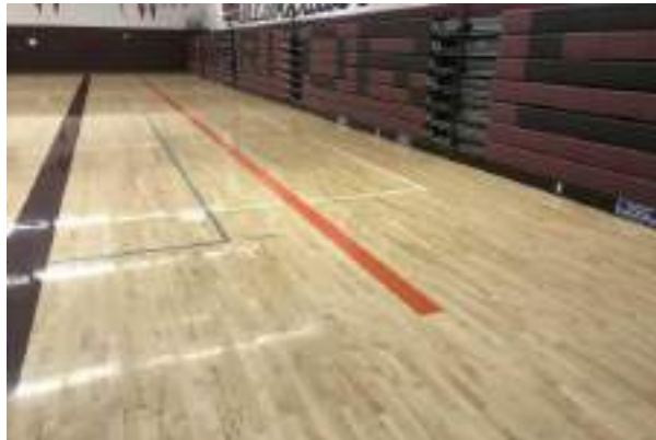
#21 014 GYMNASIUM, INTERIOR FLOOR FINISH, MAPLE SPORTS FLOOR
