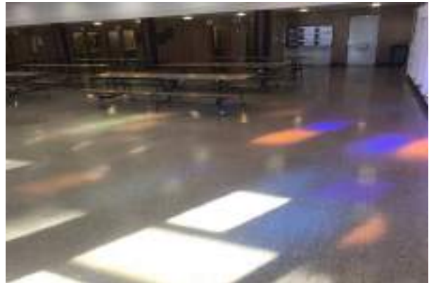
#22 015 CAFETERIA, INTERIOR FLOOR FINISH, CERAMIC TILE
