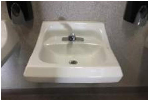
#29 SINK/LAVATORY, WALL-HUNG, ENAMELED STEEL
