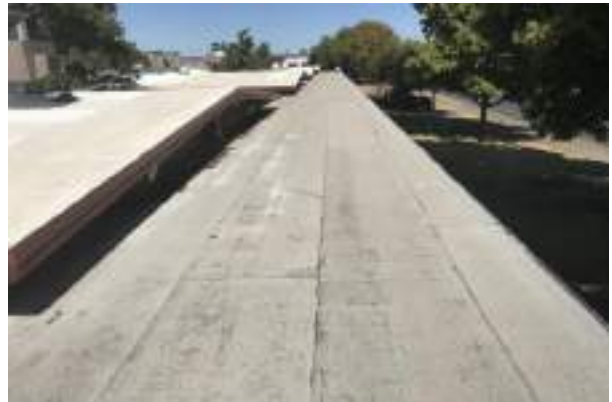
#16 SITE, COVERED WALKWAY ROOF, MODIFIED BITUMINOUS
