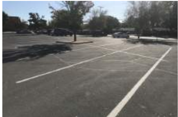
#58 PARKING LOTS, ASPHALT PAVEMENT
