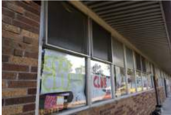
#7 C WING TO F WING, STOREFRONT, METAL-FRAMED WINDOWS
