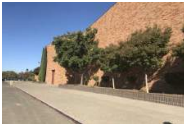
#11 16A AUDITORIUM, EXTERIOR WALL, BRICK, 1-2 STORIES
