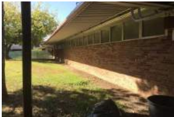
#9 C WING TO F WING, EXTERIOR WALL, BRICK, 1-2 STORIES
