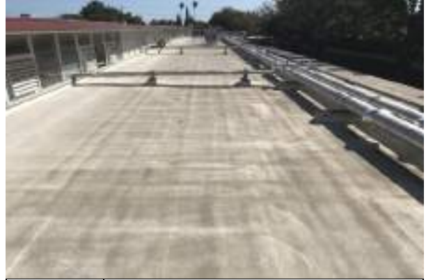
#14 011 S WING W ROOF, SINGLE-PLY TPO/PVC MEMBRANE
