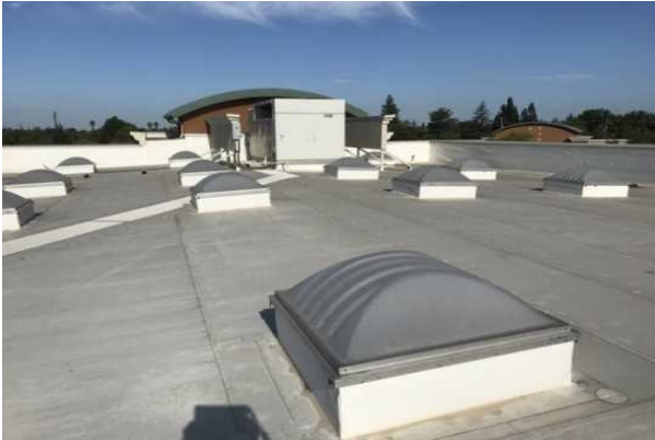
#13 SINGLE PLY ROOFING
