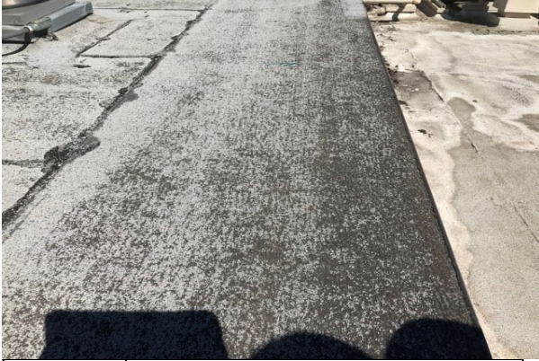
#19 ROOF, MODIFIED BITUMINOUS
