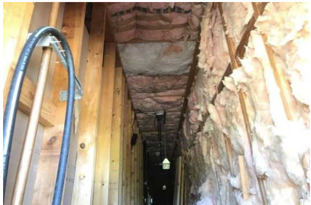
#12 STRUCTURE AND INSULATION, P07
