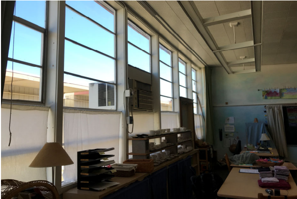
#39 BUILDING P01 WINDOWS AND AIR CONDITIONER
