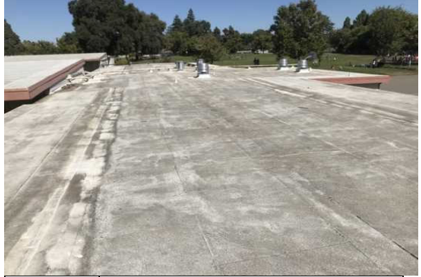
#20 ROOF AT THE COVERED WALKWAY
