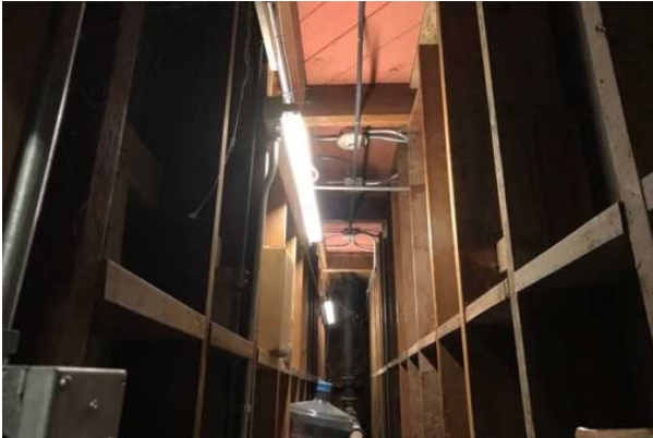
#13 PERMANENT BUILDING STRUCTURE
