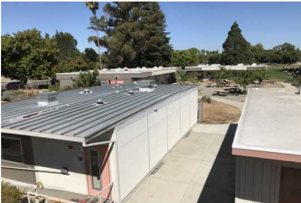
#21 P06 AND P02-3-4 ROOFS
