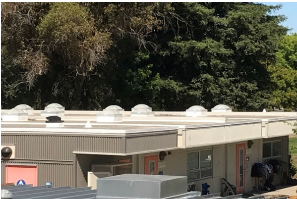
#17 ROOF, SINGLE-PLY TPO/PVC MEMBRANE, BUILDINGS P07-8
