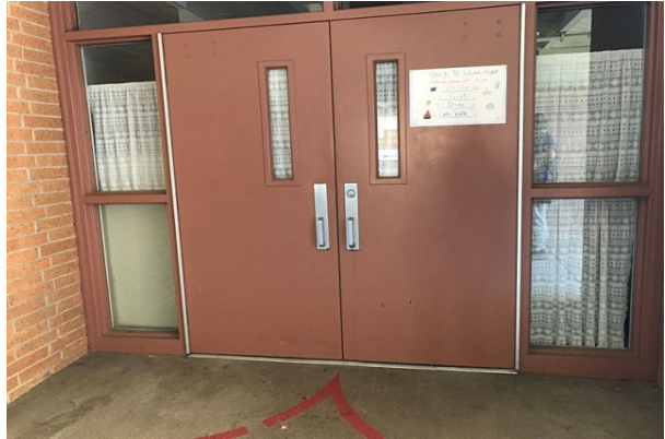
#14 OFFICE ENTRY DOORS
