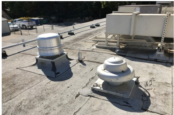
#18 ROOFING AND EQUIPMENT, BUILDING 2
