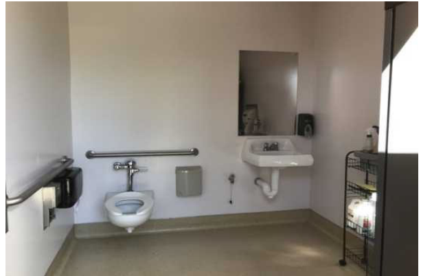
#42 MODULAR STAFF RESTROOM
