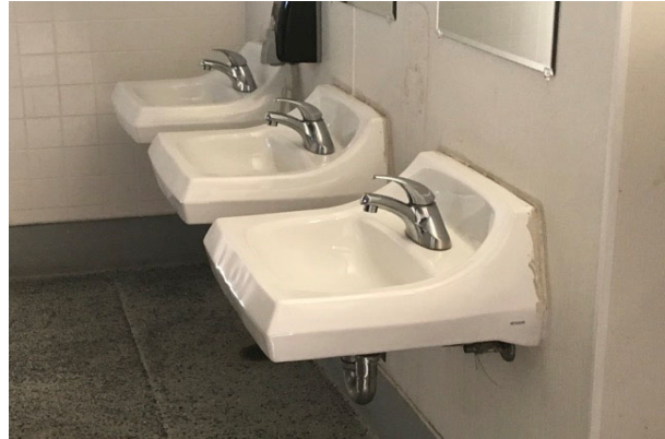
#26 D20 SINK, WALL-HUNG, VITREOUS CHINA
