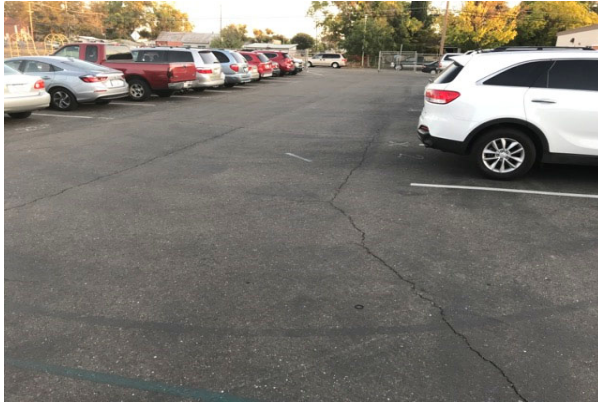
#55 G PARKING LOTS, ASPHALT PAVEMENT, MILL AND OVERLAY
