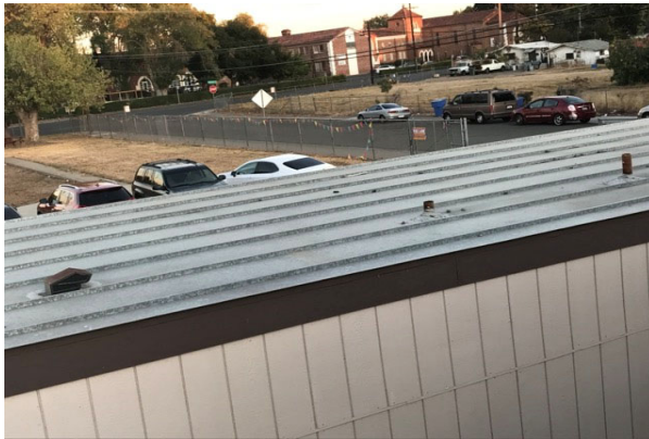
#15 B30 ROOF, METAL
