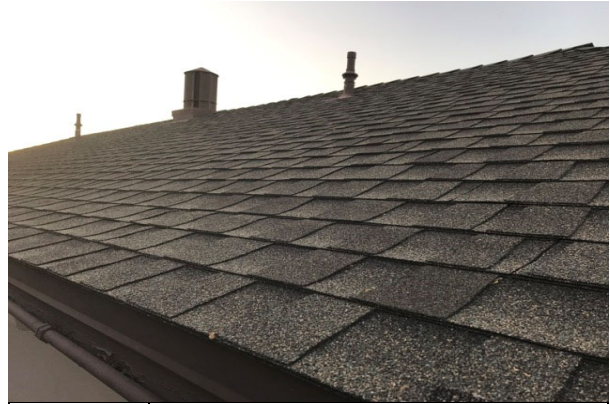
#14 B30 ROOF, ASPHALT SHINGLE
