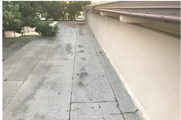
#16 B30 ROOF, MODIFIED BITUMEN
