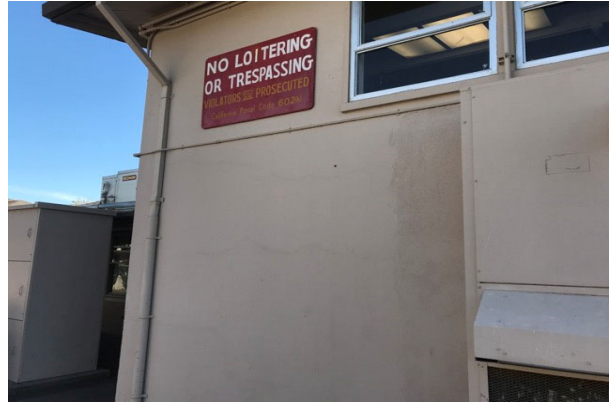
#8 B20 EXTERIOR WALL, PAINTED SURFACE
