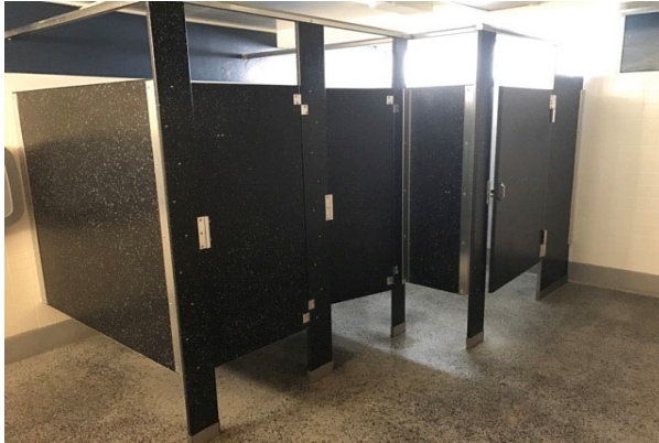
#19 C TOILET PARTITIONS
