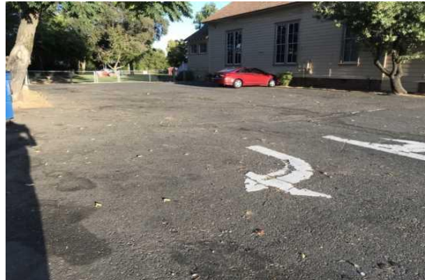
#18 PARKING LOT, ASPHALT
