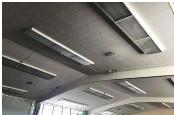
#48 HARD TILE CEILING
