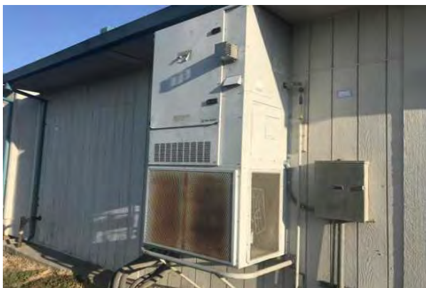
#65 WALL-MOUNTED GAS PACKAGE UNIT
