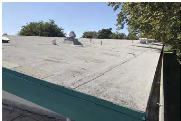
#34 002 MODIFIED BITUMINOUS ROOF
