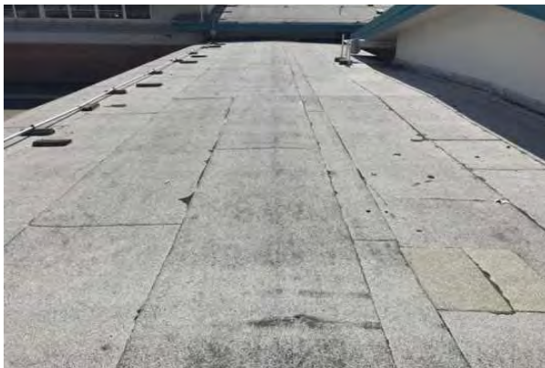
#35 COVERED WALKWAY MODIFIED BITUMINOUS ROOF
