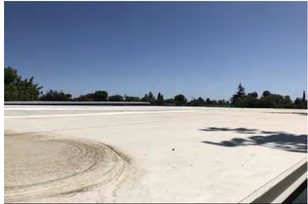
#38 1991 PORTABLE TPO/PVC MEMBRANE ROOF
