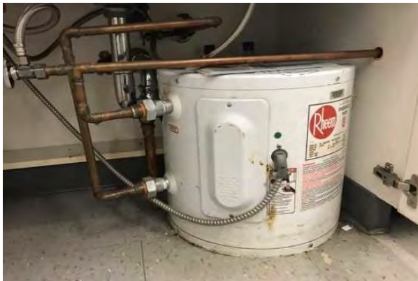
#57 ELECTRIC WATER HEATER
