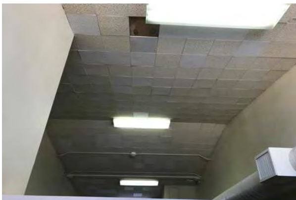
#47 HARD TILE CEILING
