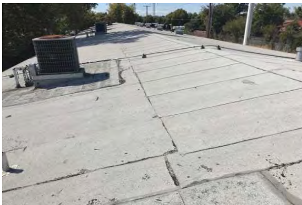
#33 001 MODIFIED BITUMINOUS ROOF
