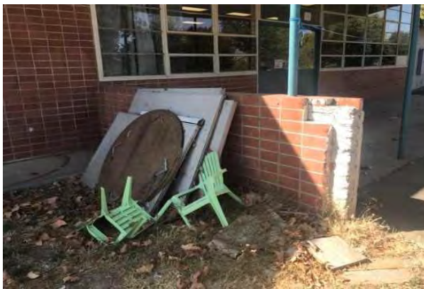
#27 DAMAGED BRICK
