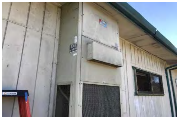
#66 WALL-MOUNTED HEAT PUMP
