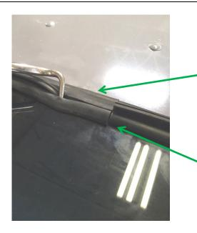
Once you get glass fully inserted into gasket, you will need to use the gasket tool to push the locking flap into the gasket around the whole window. This locks the window into place.
