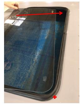
Start glass installation by sliding in a corner into gasket (+) and pivoting other side into opposing corner.
