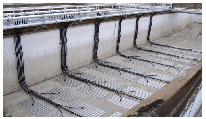
The **PB Equipment™ Bosman® Plate Aerator™** fine bubble aeration in activated sludge wastewater treatment has unquestionable advantages over coarse and medium bubble aeration in respect to oxygen transfer efficiency and therefore lower power consumption. Fine bubble aeration will pay for itself in power costs after only a few years of operation due to this high efficiency.
