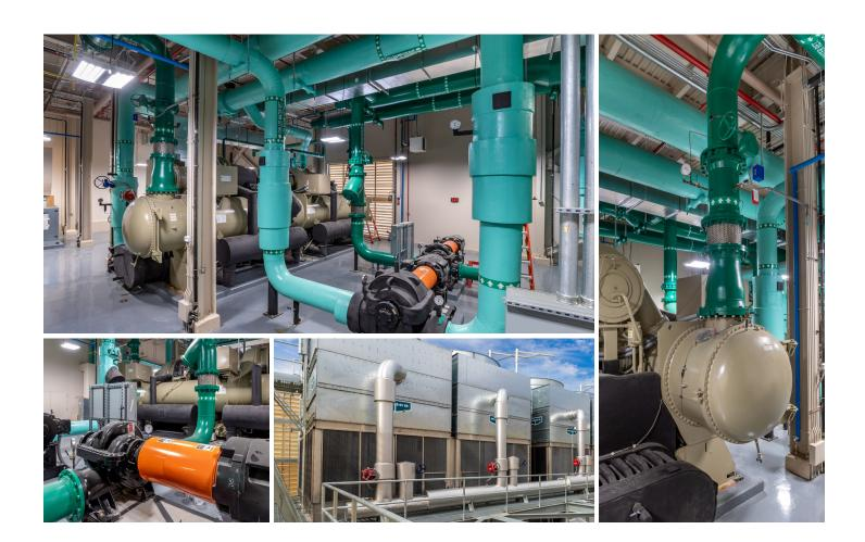
Construction of a new two story steel framed building which is an addition to the North Energy Plant for the installation of one 3,000 ton chiller, cooling tower, pumps and the installation of chilled water distribution piping. An extensive underground piping installation, as part of USC's expansion of the chilled water distribution loop, was included in this project. The underground piping included a large, horizontal, directional bore under Blossom Street in downtown Columbia.
