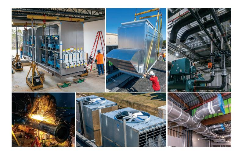
HVAC installation at the new 120,000 sq. ft. Forensics Lab at the South Carolina State Law Enforcement Division (SLED) in Columbia, SC. The project comfort air is handled by means of two 500-ton chillers, cooling towers, boilers
