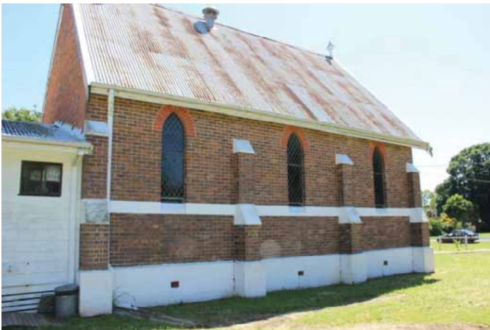
Figure D4. The side elevations of the 1908 brick church are divided into three bays by four buttresses with rendered coping. Pointed-arch windows have diaper-pattern leadlight of coloured glass, with red-brick voussoirs above. Note the lapped galvanised corrugated iron roof with original ventilators.
