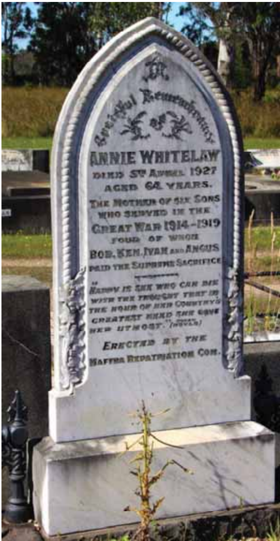
Figure D1. View of the front of the gothic memorial headstone and base, both made of marble with hand carving and lead lettering.
