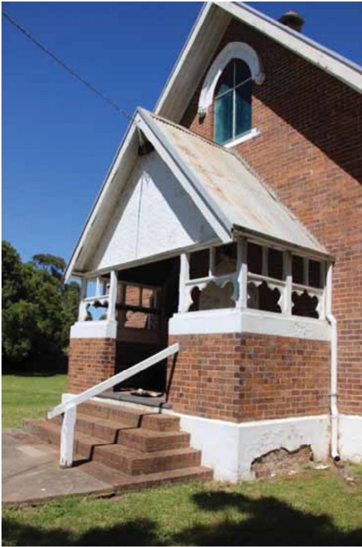
Figure D2. The entrance porch with the pressed metal cladding to the gabled end imitating a rough-cast render, timber tracery and brick balustrade. Note the damp damage to the render of the plinth.
