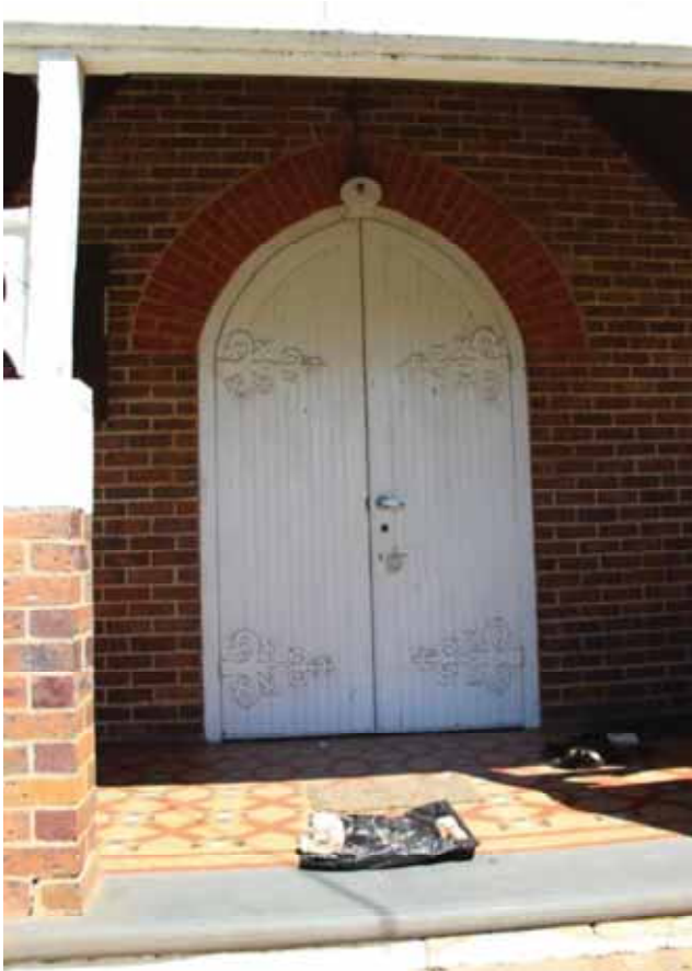
Figure D3. The entrance porch has the original tessellated tile floor. The entrance doors are pointed arched double timber ledged doors, framed by a slightly pointed-arch of radiating tuck pointed red-brick voussoirs above.
