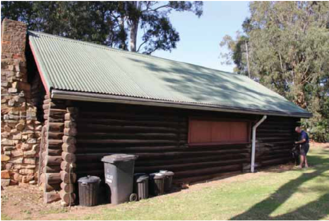
Figure D3. The north elevation with its wide timber-framed window with its original timber shutters (like the main elevation).
