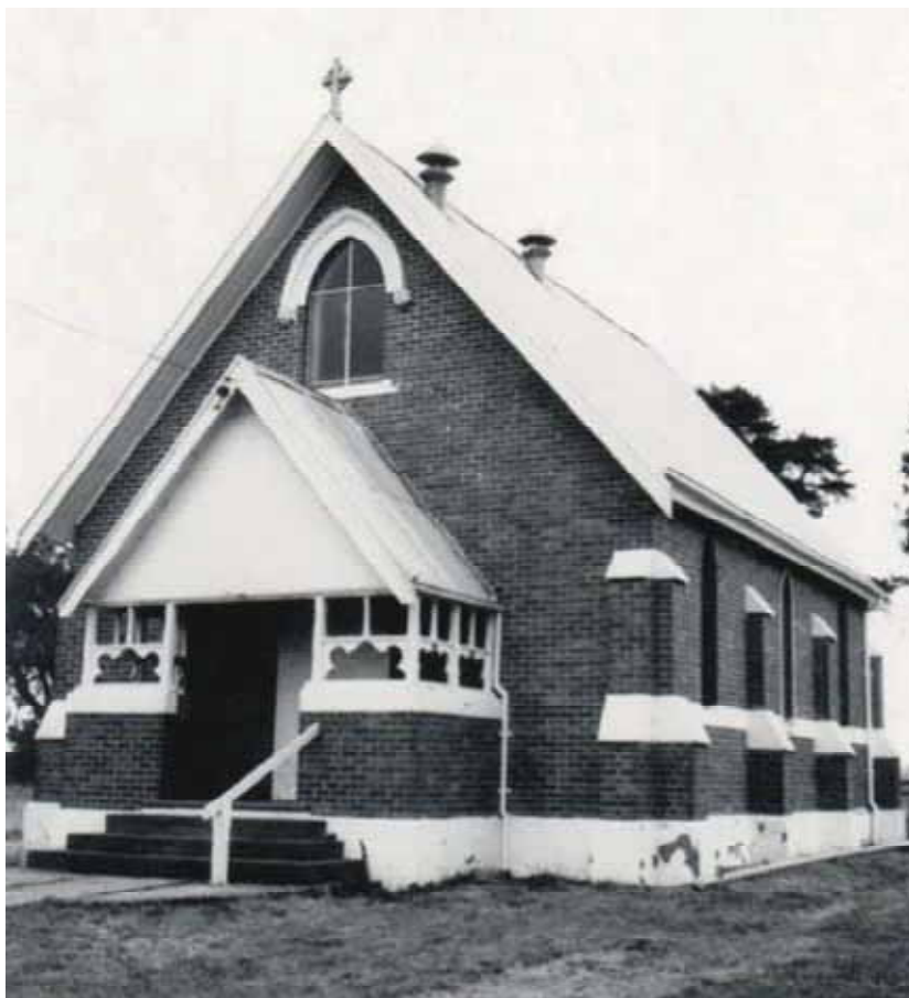
Figure H2. The facade and north elevation of the church in 1976, with the entrance porch and its plain gabled-end and single timber balustrade to the steps (MDHS, ID. P02783VMFF 1976).
