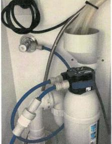
A ventilated odour trap / s-bend with an open tun-dish must be provided
