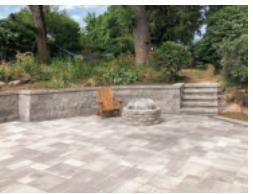
RETAINING WALLS & FIREPITS
