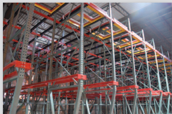
Hybrid system with push back above drive in
