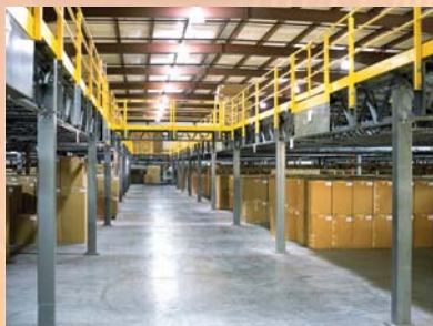
Warehouse Mezzanine with Walkway Bridge
