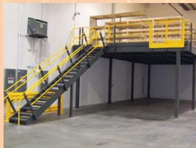
Small Mezzanine with Stair and Swing Gate
