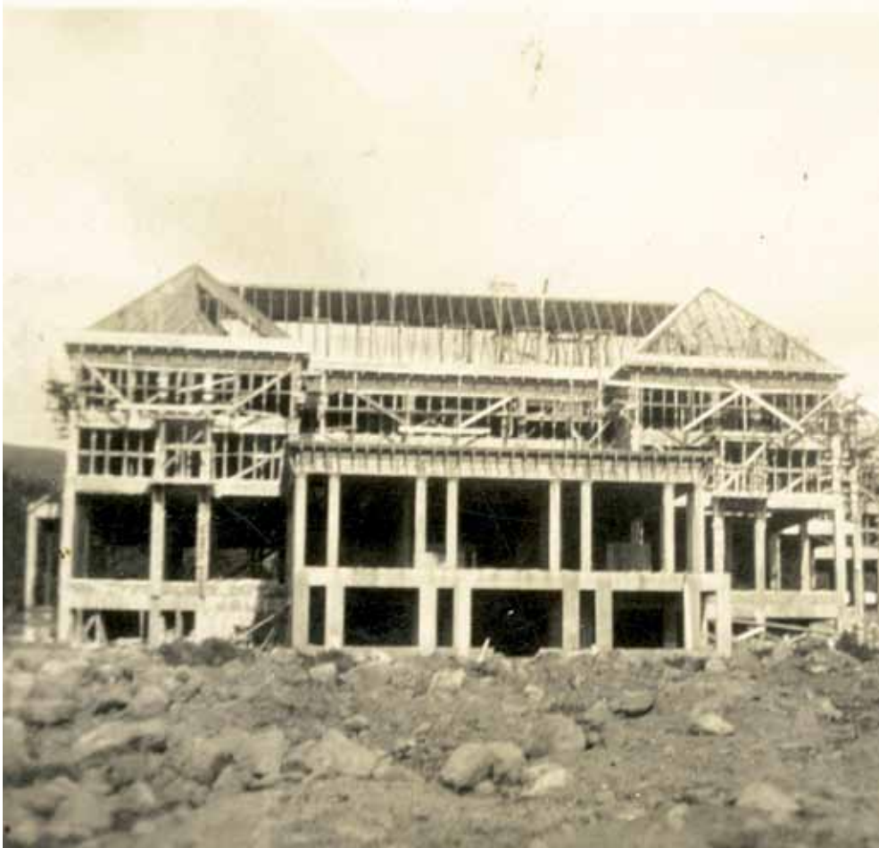
The Chateau under construction 1929. Photo: Ian Matheson City Archives .
