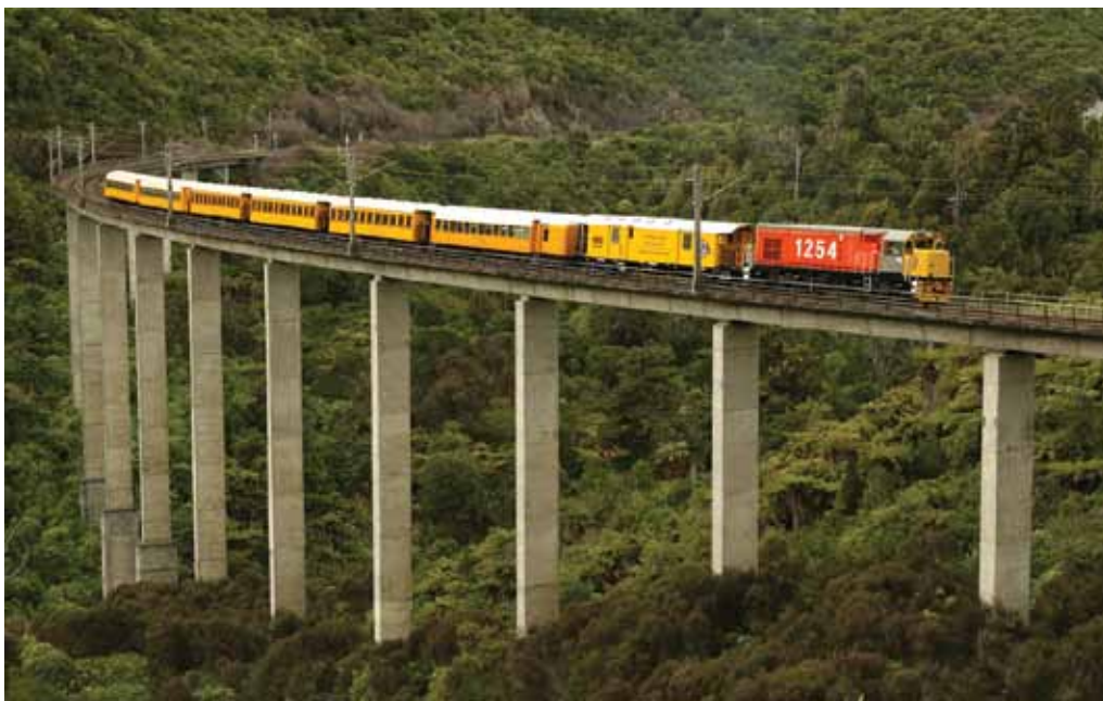
A Glenbrook Vintage train crosses the Hapuawhenua Viaduct.
