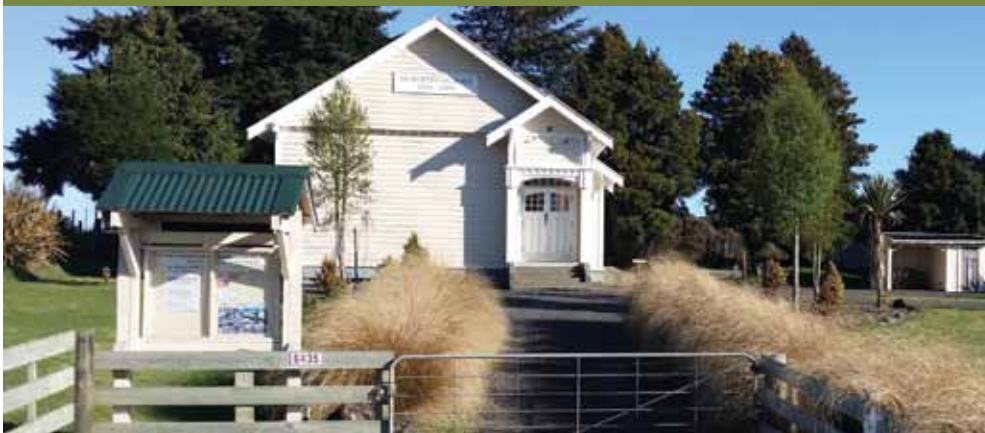
Community Hall Repairs & Maintenance Fund
