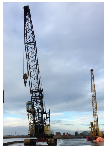
Crawler Crane fitted with CSP-W402 Camera attached to the Cranes Hook
