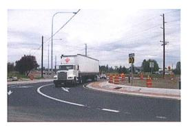
the oversize vehicle can ride up on the truck apron so the truck can easily complete the turn, while the raised portion of concrete discourages use by smaller vehicles.
