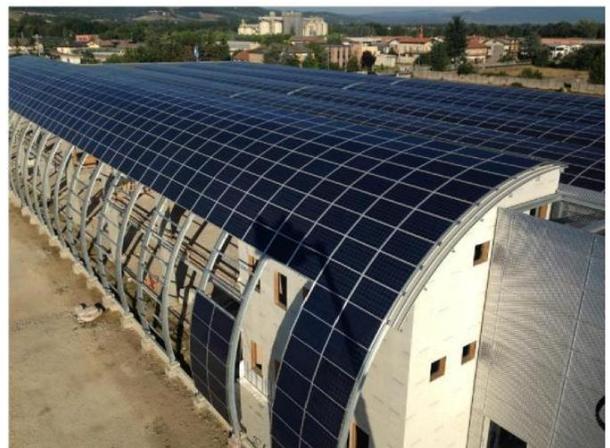
Tigo’s panel-level MPPT corrects for mismatch caused by the curved façade and shade cast by nearby light poles.
