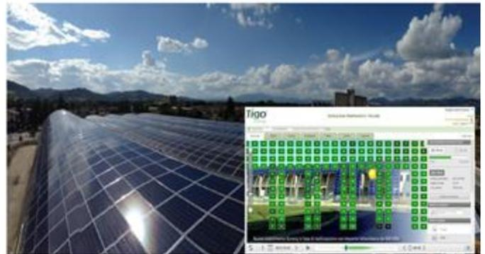
Panel-level monitoring helped in the commissioning process, which is extremely important when modules are difficult to access, such as in vertical façades.
