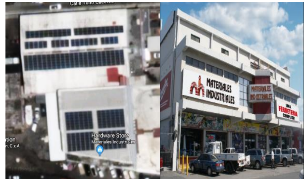
A rooftop view of the 132.4kW PV system with 420 retrofitted modules in Dominican Republic.
