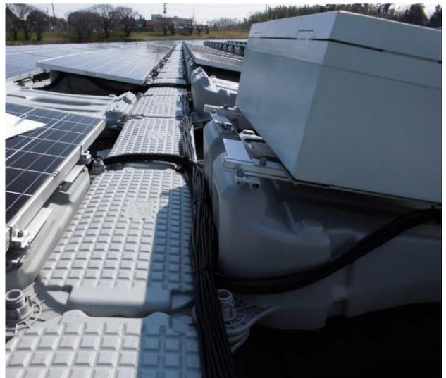
Tigo TS4, whether PV module integrated or add-on, are non-metallic and do not require any special grounding. Therefore, they simplify the installation by providing additional features with practically no additional work when mounting.
