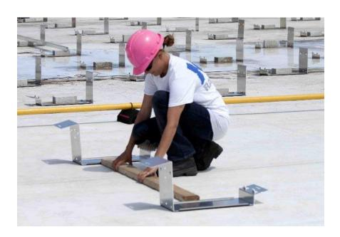
Figure 4 - Use of Spacer Sticks to Aid Placement
