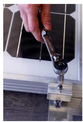
Fig. 13 - Use Torque Wrench
