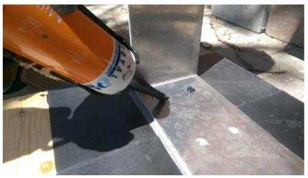
Figure 5 - Step 6: Apply LPS sealant on/in predrilled holes
