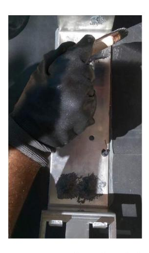
Figure 7 - Step 8: H.E.R Sealant painted on screw heads
