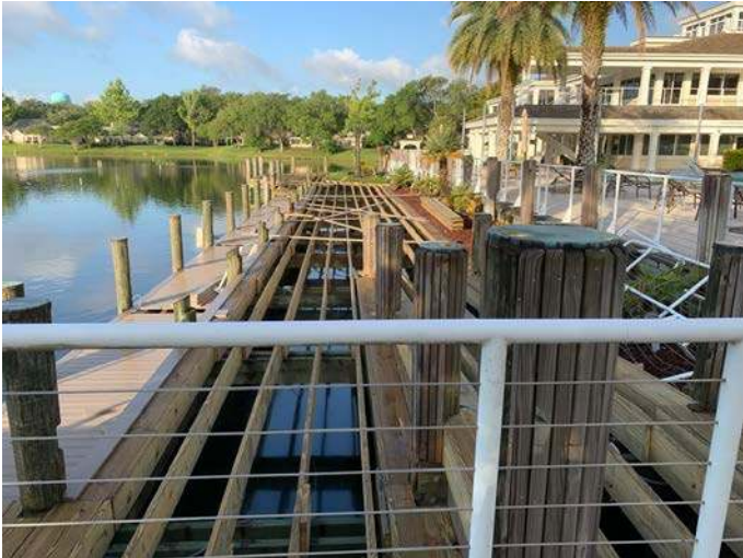
The deck in the dock area closest to the pool has been partially rebuilt.
