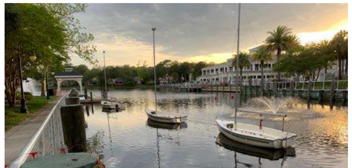
The sailboats, which had to be moved while the dock is being rebuilt, have been secured in two different ways on the 1000 Building side of the lake.
