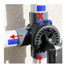
1. Depending on how complex the system you may have valves in place to direct the water flow to different lines of the pool system. This will allow you to control the flow for different reasons. It is extremely important that the valves are open to correct way otherwise it can result in damaged equipment, burst pipes & more.
