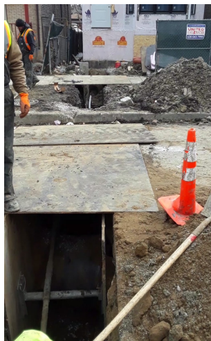
Figure ES.6.1: Open Cut Service Line Installation
