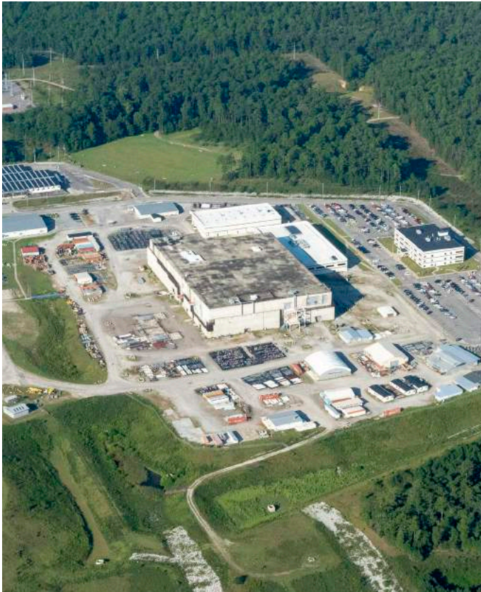
Sunk by huge cost overruns and mismanagement, the MOX facility is the site for unprecedented plutonium pit production. Photo: High Flyer © 2020
