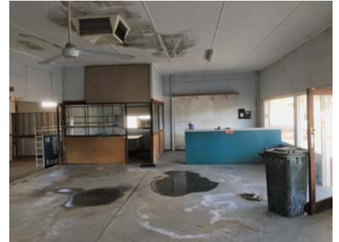
The long unoccupied Koorda store before renovations.
