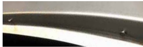
Deck filler rivits are installed.
