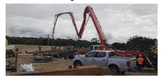
Project is on schedule, with stage 1 nearing completion. The bridge replacement reached a major milestone with the concrete deck being poured.
