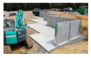
The saw tooth bays are complete and works on the road sealing have commenced. Waiting on fill materials testing results as per EPA regulations before final construction commences.
