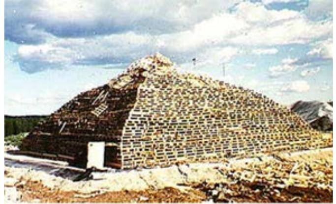
Figure 6.1: Leachate evaporation pyramid at Hogbytorp landfill, Sweden
