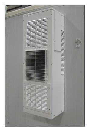
The primary purpose of the **Green HVAC** is to save energy while maintaining a well regulated environment inside the shelter. This is done by monitoring the inside and outside environment and intelligently choosing the least expensive mode of operation, while limiting the inside environment to a user settable temperature range.
