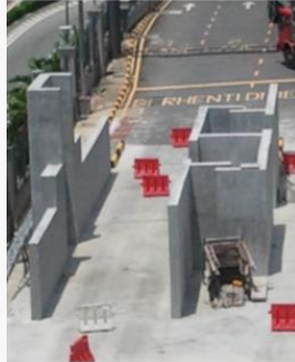
Example of Construction of Radiation Shielding Walls to house one Scanning Portal
