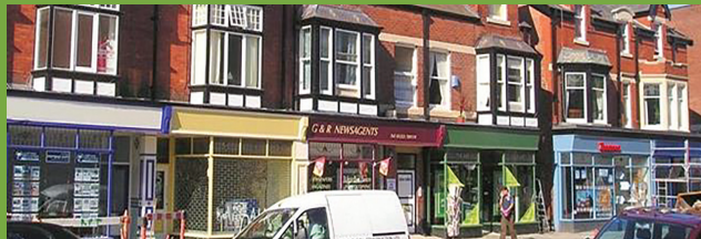
Example of shop front reinstatement with grant aid in St Anne's delivered by the Regeneration Team and the building owners
