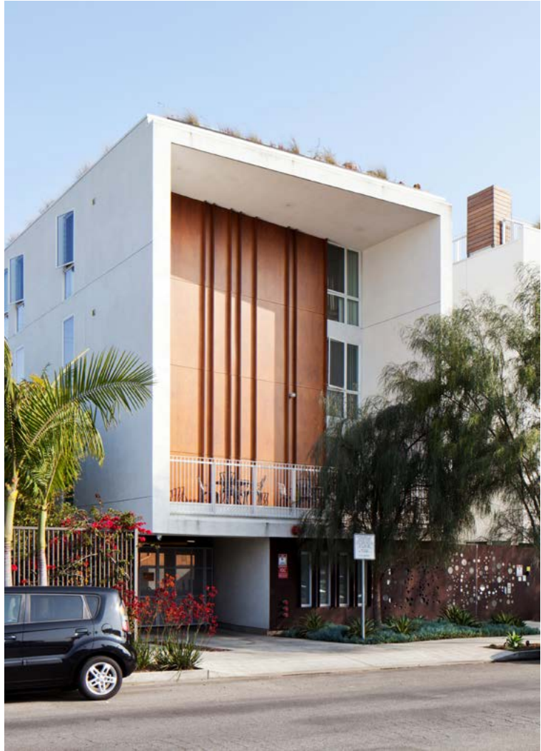
Product: Facade / Woods: Copper and Antra Gateway Apartments, by Brooks+Scarpa Architects (Marina Del Rey, CA, USA)
