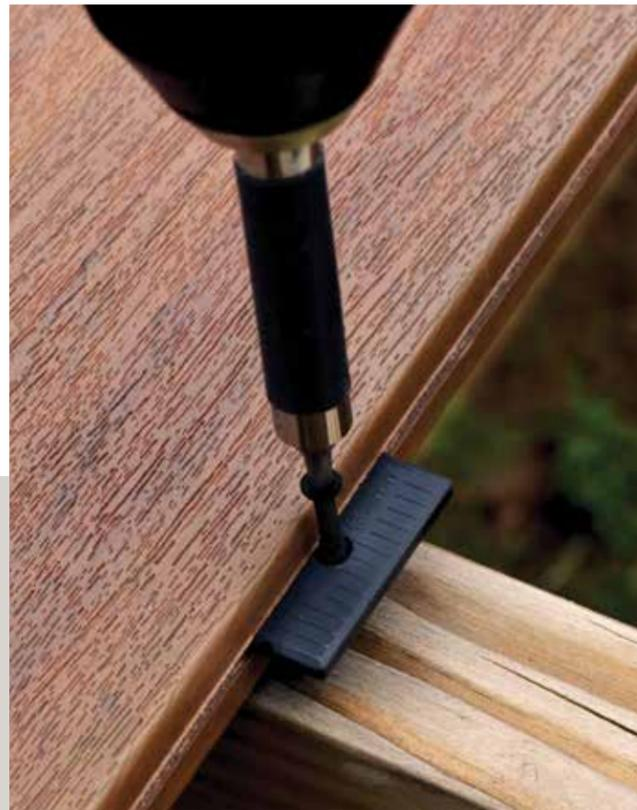
For the Phantom universal fastener, the clip is installed into the groove. Then, a screw is driven straight down into the joist (90-degree angle).
