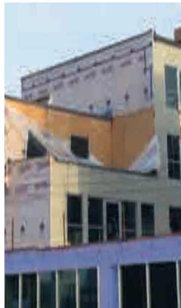
It is common for housewraps to be damaged and require rework after a wind event.
