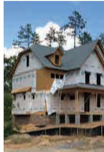
It is common for housewraps to be damaged and require rework after a wind event.
