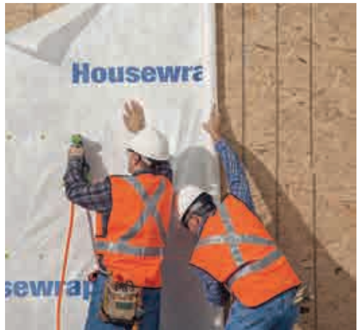
Traditional housewrap systems are often clumsy and require two installers, making multistory applications and windy environments especially tricky.
