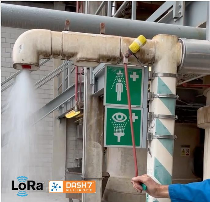
Having the **real time position** of emergency showers available will potentially **increase emergency responds time**. Following local regulations, emergency showers need to be regularly opened. This is now **automatically time stamped**, logged and can be used to monitor whether this has been done. Additionally, the usage of a shower is logged and can be used to **automatically trigger an incident report**. Incident reporting is key to increase safety by learning from what went wrong.
