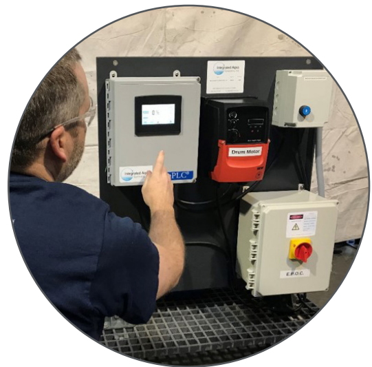
AquaPLC™ touchscreen controller is fully programmable for Intelligent, Basic or Continuous drum operation.
