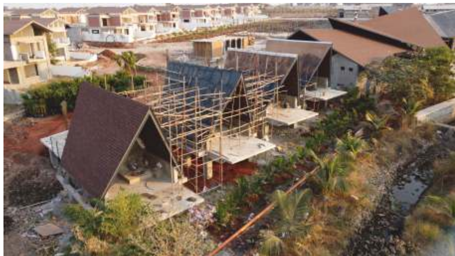
Rurban Hive - Shingles work completed
