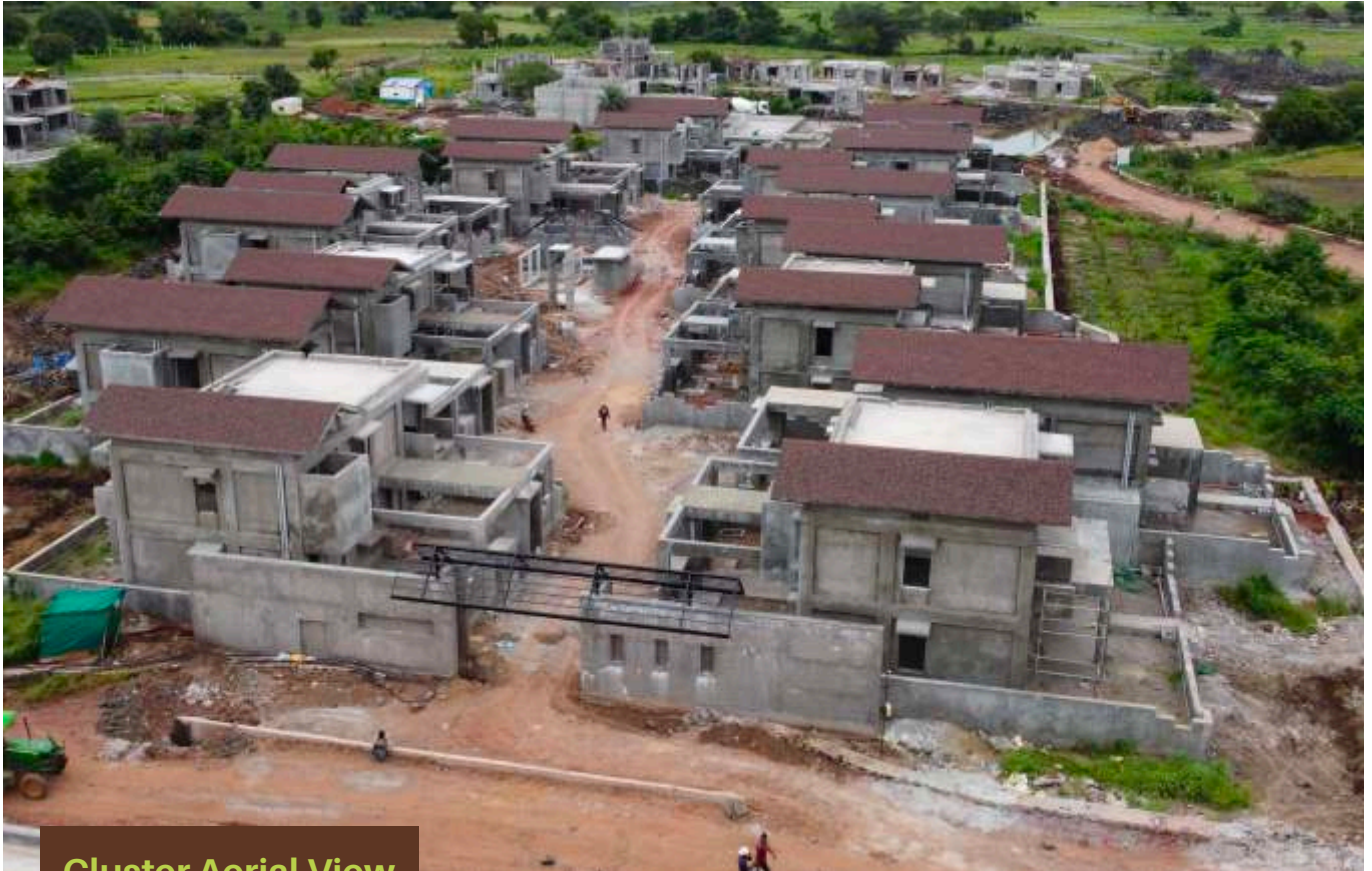
Cluster Aerial View
