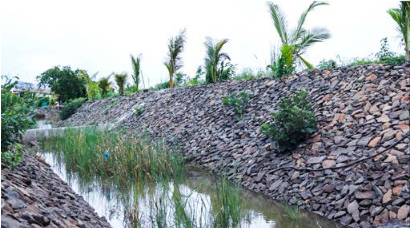
Natural water stream with check dams
