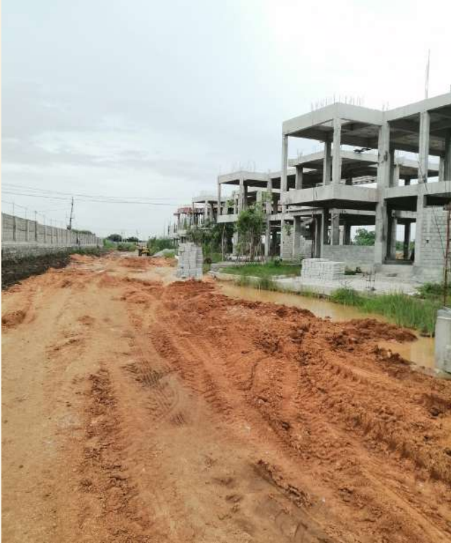
Front side view of the West Facing Villas
