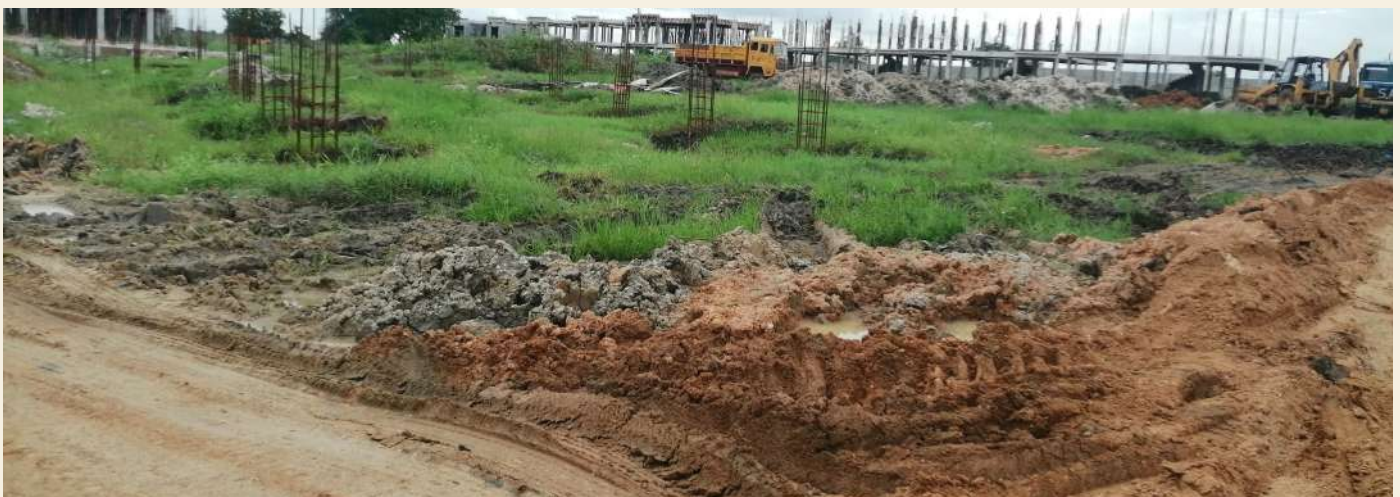
Footing work in progress at the Club House Area
