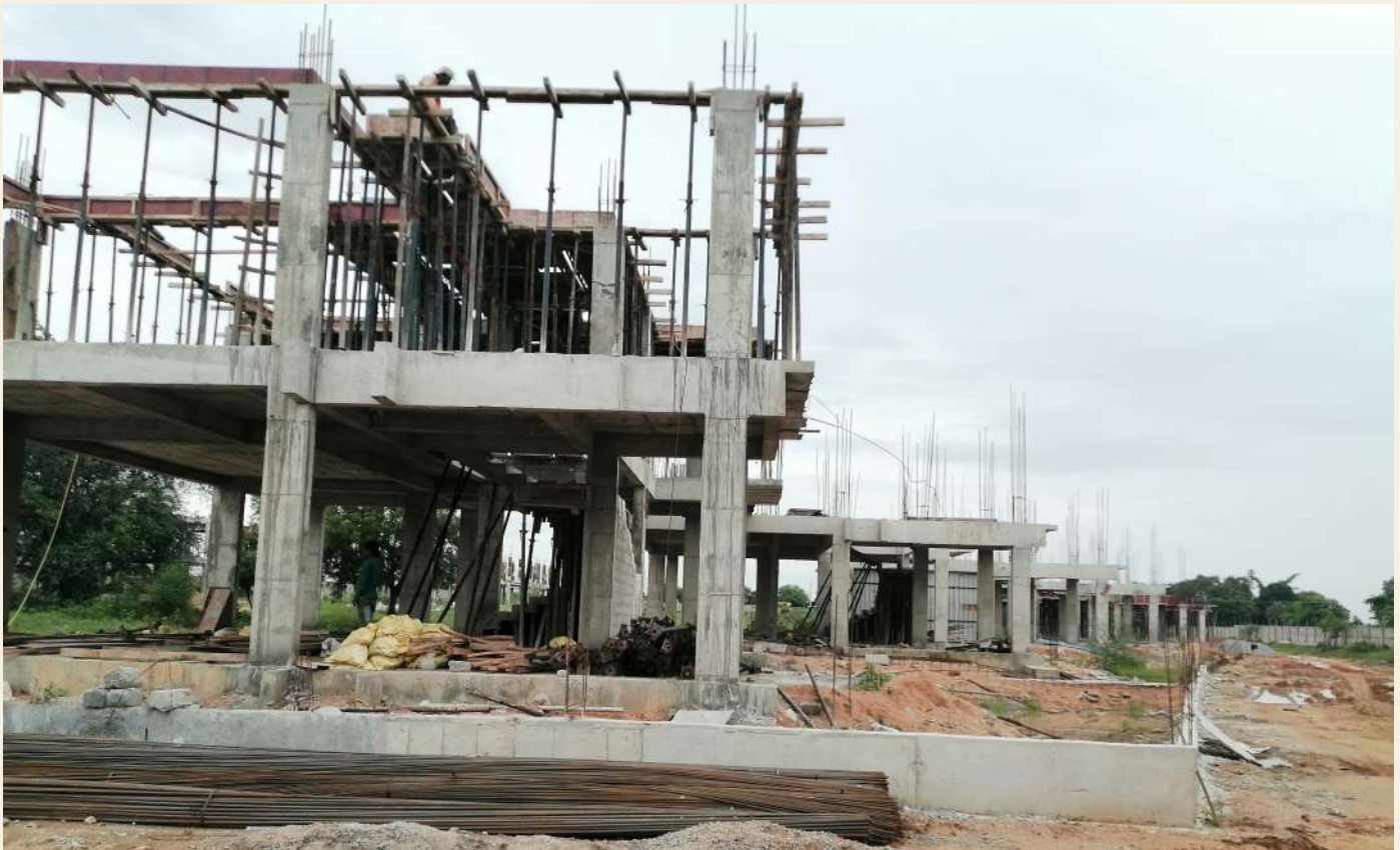
East Facing Villas ready for PCC Flooring after first-floor slab completion
