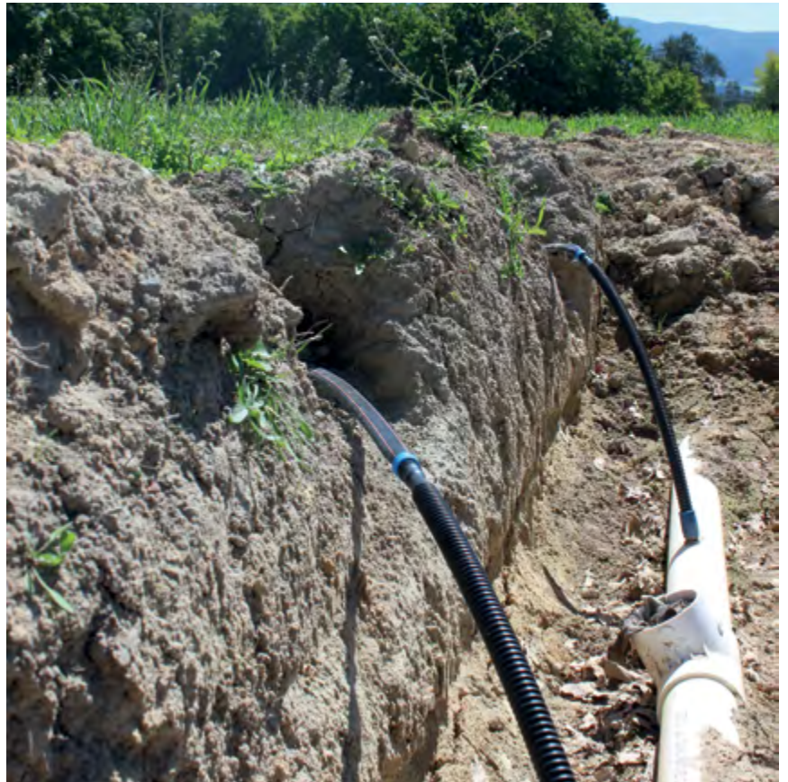
Sub-surface drip irrigation installed.
