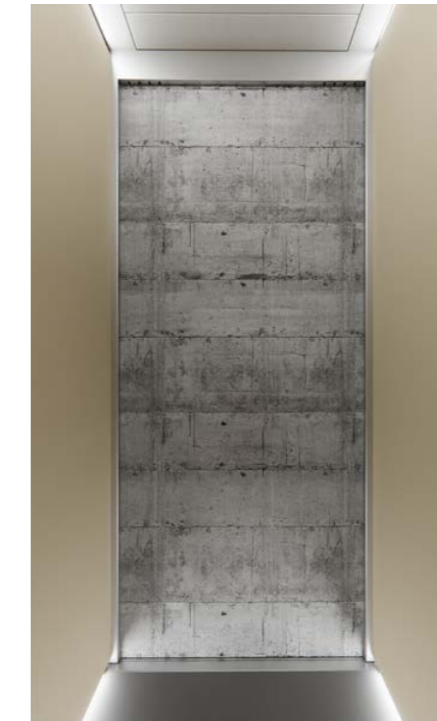
BEFORE WITH EXPOSED MASONRY WORK
