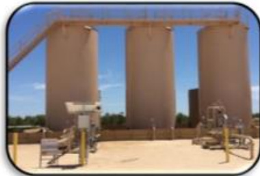
Centralized Crude Gathering Tanks at Reagan Truck Station
