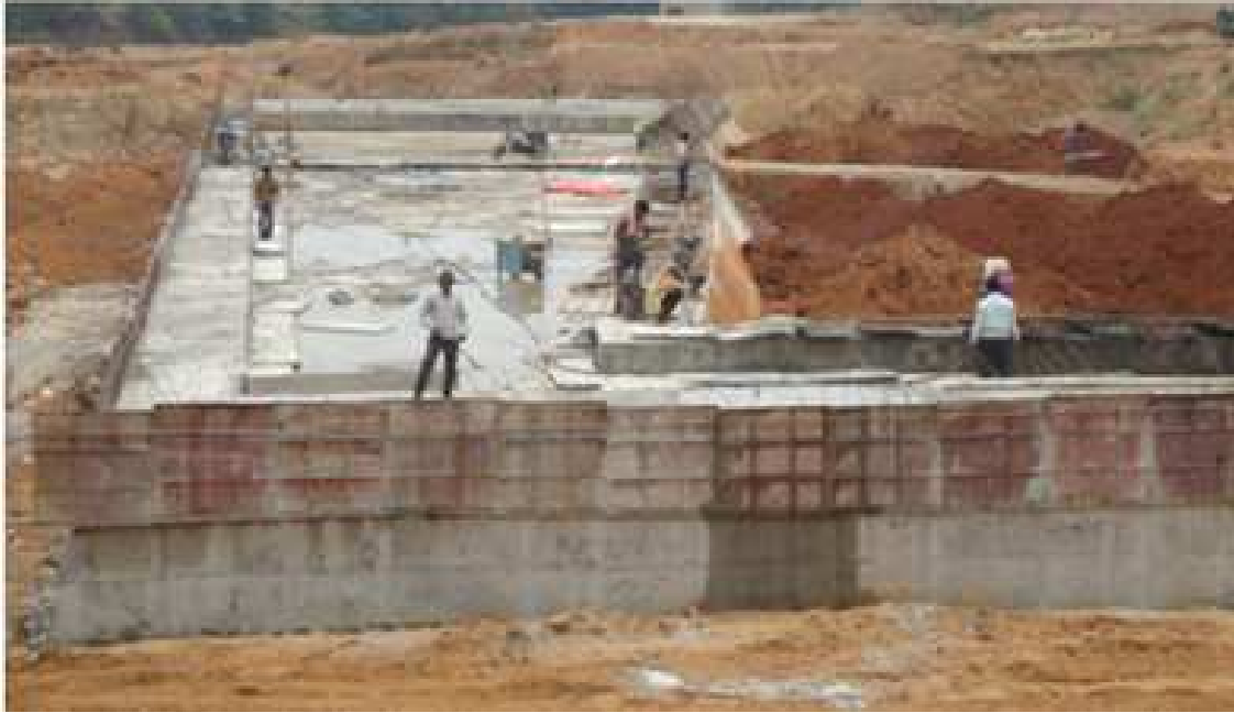
View of U/S Right Wing Wall
