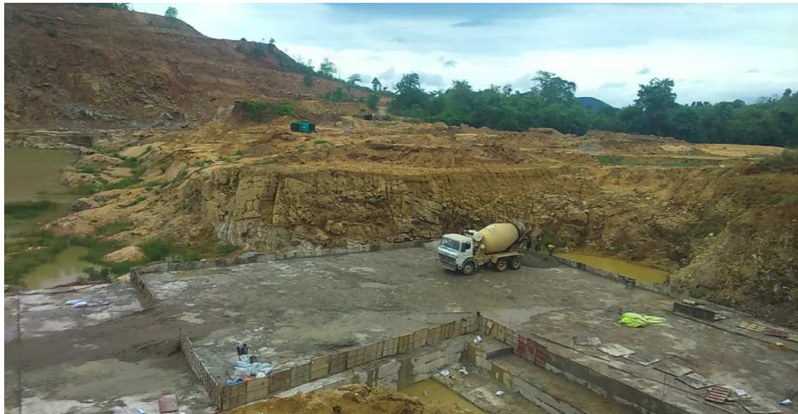
View of D/S Right Wing Wall
